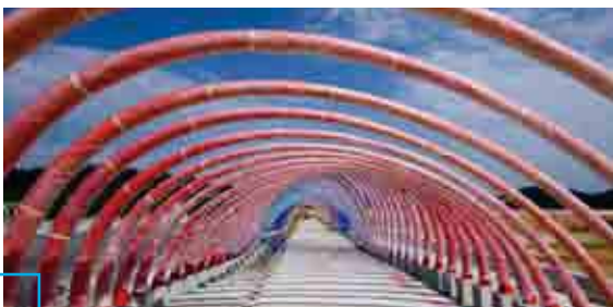
Picture: Rainbow Bridge at Elmina, Denai Alam, Shah Alam completed by G-Cast UHPC
