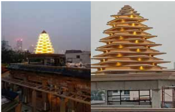
Picture: Shree Lakshmi Narayan Temple located at Jalan Kasipillay, Kampung Kasipillay, Kuala Lumpur – Temple dome tower structure construction using UHPC with high detailing finishing and design
