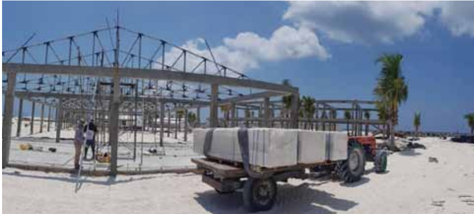
Picture: Starken AAC supplies the AAC panels to 4 star Maniyafaru Resort in Maldives. The AAC panels are used as the wall panels for 262 villas and many of the ancillary buildings in the resort.
