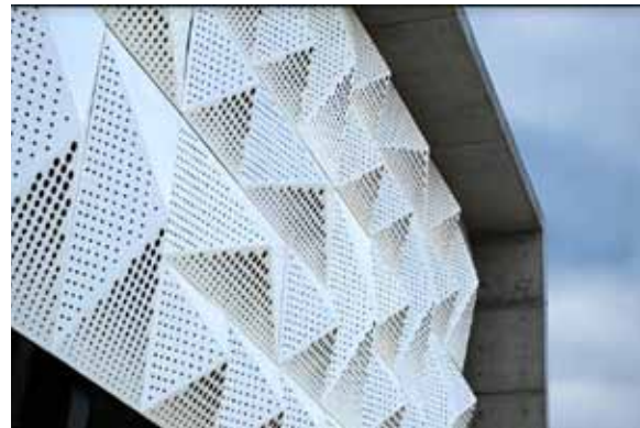
Picture: Very light, thin 3D decorative panels constructed using Fibre Reinforced Polymer ("FRP") at SP Setia Temasya Sales Gallery completed by G-Cast UHPC
