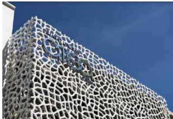
Picture: ATSA Corporate Office located at Taman Tun Dr Ismail, Kuala Lumpur – Façade cladding customisation of unlimited pattern possibilities tailored to Architects and clients requirement, completed by G-Cast UHPC
