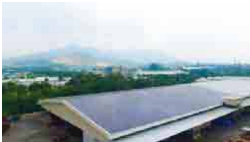
Metex Steel Factory (1MW)
